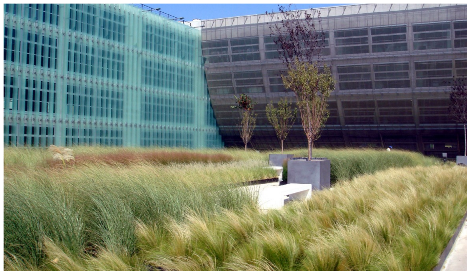
The roof garden of the Shop & Trade Office Building about a year after its completion.
