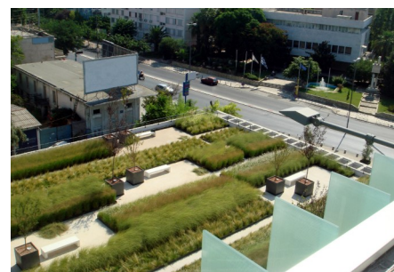
The system build-up based on Floradrain® FD 60 protects the waterproofing and contributes to the thermal insulation of the building.
